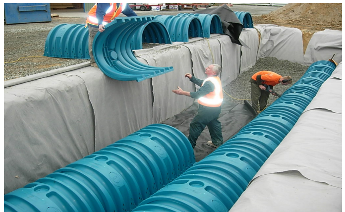
Quick and easy installation of arches
