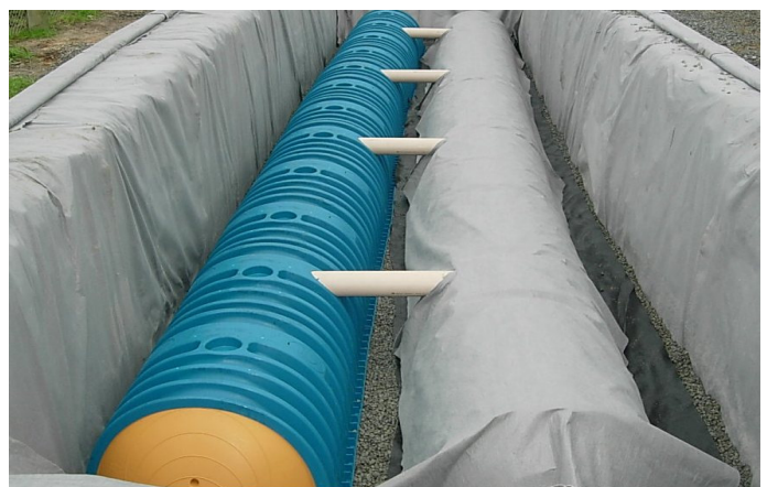
EcoAid arches ready for backfill
